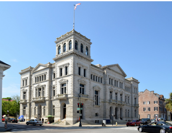
US COURTHOUSE AND POST OFFICE, CHARLESTON, SC, A SECTION 106 SUCCESS STORY (WIKIMEDIA COMMONS)
